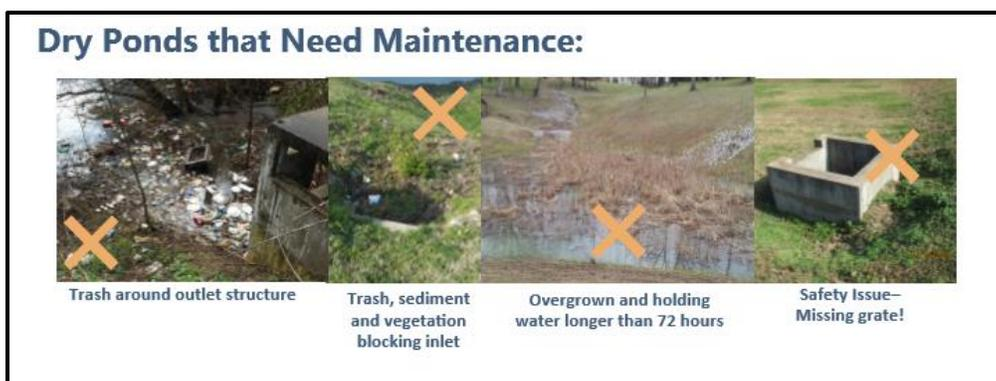
**To ensure that a detention basin is working properly, it is important that it is properly and routinely maintained.** Examples of detention basins in need of maintenance, as provided by Nashville Metro Water Services, can be seen above.
