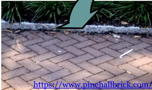
Permeable pavers are susceptible to clogging by organic matter, sediment, and other debris. They therefore need to be occasionally inspected, cleaned, and maintained to ensure desired infiltration rates.
