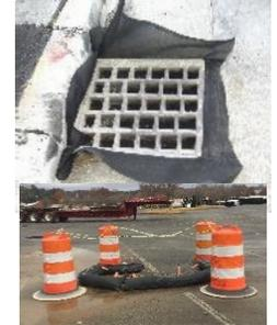
**Inlet protection:** Protect storm drains by lining grates with filter fabric, or surround with gravel bags.
