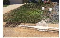
**Concrete washout:** Contain excess concrete, mixing water, or wash water from construction activities. Do not allow chemicals to runoff into storm drains, and waterways.
