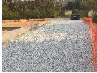
**Sediment traps:** Used to capture sediment and keep it on site. Ensure proper installation by entrenching a portion of the material underground, and securing it in place. Do not use straw bales to capture sediment.
